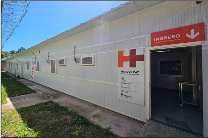
FIGURE 4. MHS federal complex rehabilitation center for young adults, Marcos Paz, Buenos Aires.
