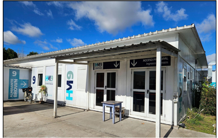
FIGURE 6. MHS No. 9, Almirante Brown, Buenos Aires. A prefab module to complement an existing center.
